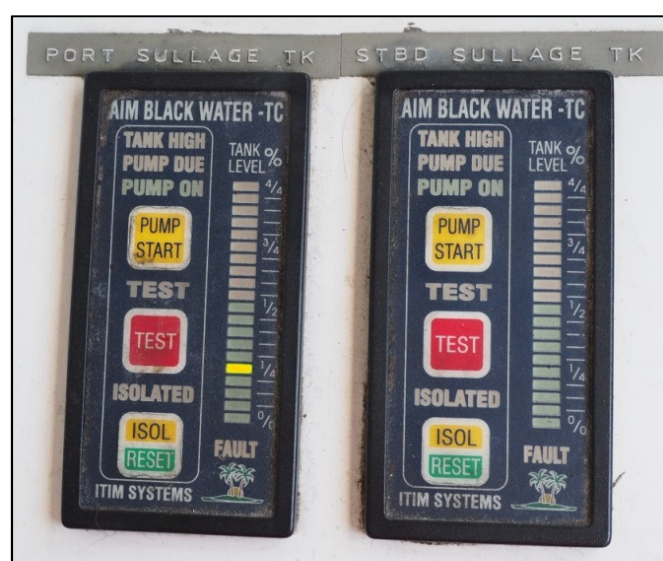
Figure 24: Sullage tank indicator panel with pump start switch
