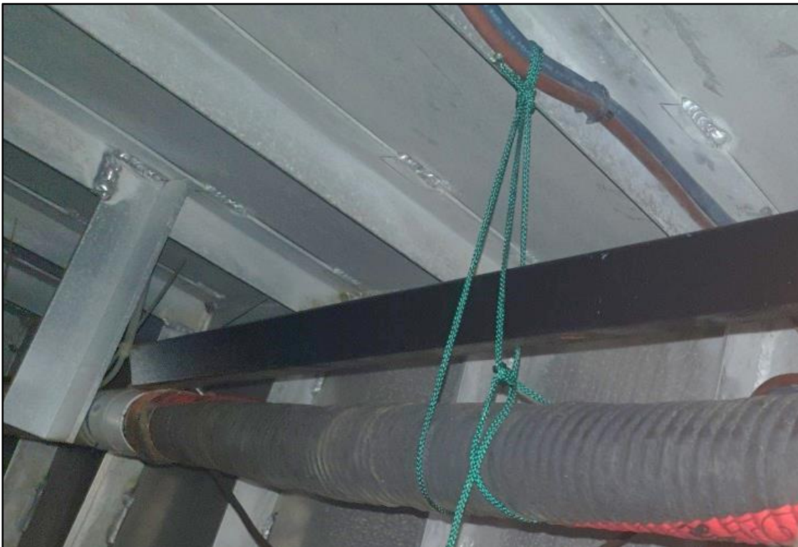
Figure 12: Chord securing rubber hose fitted to vent line
