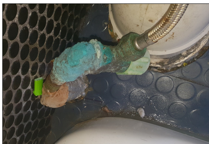
Figure 22: Water inlet valve showing blackening of chrome finish
